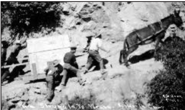
Sledding a piano to Roberts' Camp, ca. 1930. Jim Heasley is leading the mule. He wrote on the reverse of the photo "The piano had to be tuned!" E.B. Gray photo. Heasley Collection. Sierra Madre Historical Archives.
